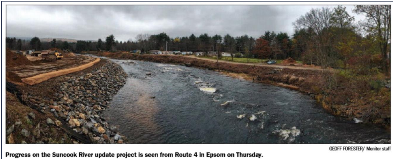
Figure 17a Suncook Channel Stabilization Project
